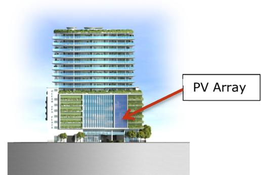
It is presently not acceptable to install electricity generating equipment into the Gibelec grid. However, the PV cells, electrical infrastructure and containment could be installed initially, but remain unconnected so that PV could be energised once permitted by Gibelec.
